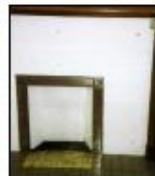
Asbestos insulating board (AIB) fire surround
